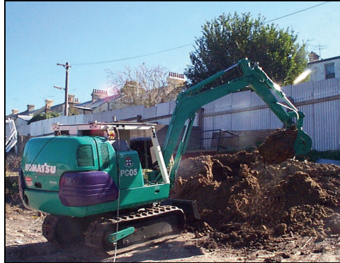
Fig. 5. the Automated excavator of the University of Sidney
