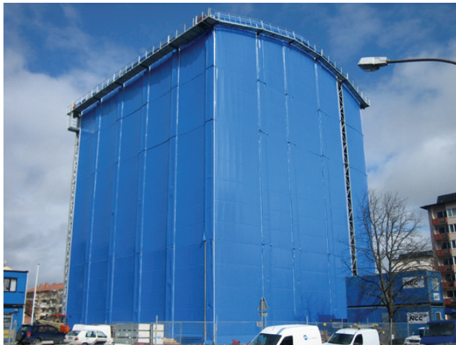
Fig. 11. On site factory of NCC Komplet
