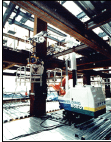
Fig. 11. WR mobile robot for column welding
