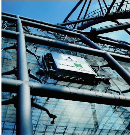
Fig. 1. Automatic Facade Cleaning System for the Vaulted Glass Hall of the Leipzig Trade Fair ( Fraunhofer FhG )
