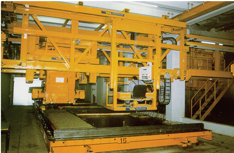
Fig. 4. Teleoperated concrete distribution
